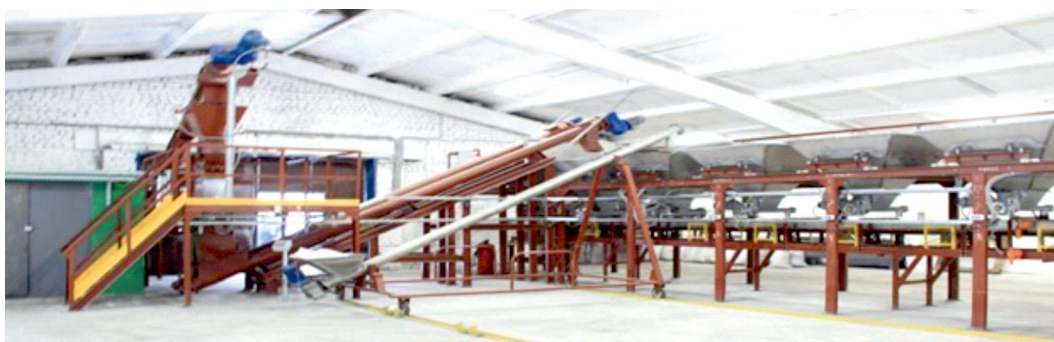
Poultry house sorbent production plant
